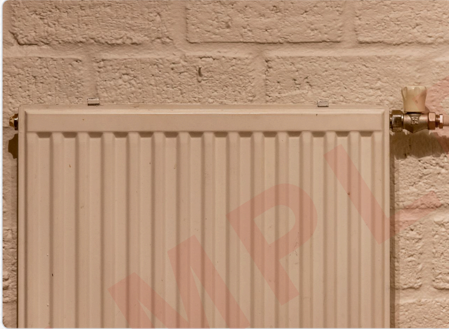
Radiator with lockshield valve
