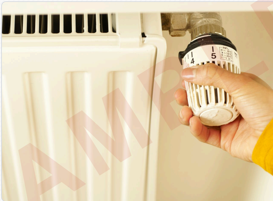
Thermostatic radiator valve
