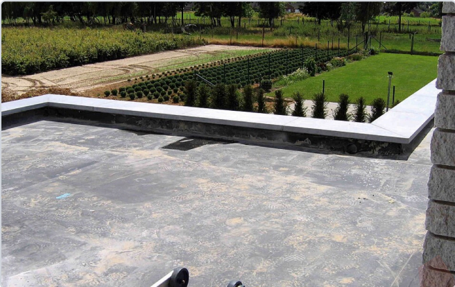
5a Rear extension: EPDM membrane bonded and in good order
