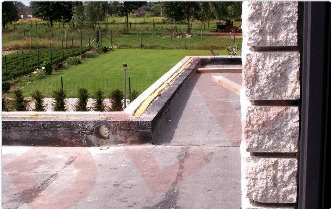
5b Scupper outlet through the upstand: clear
